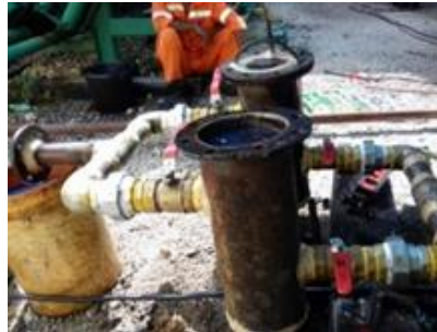
Figure 11. Fuel filter testing process
